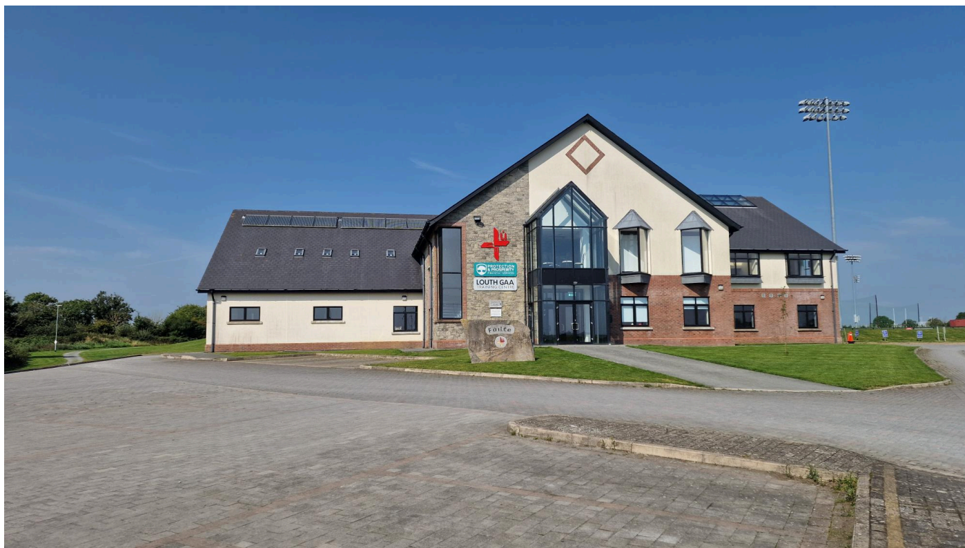
Protection and Prosperity Louth GAA Training Centre, Darver
